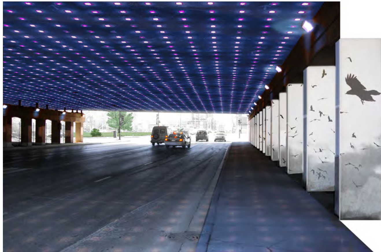
Figures 106a. and b. Photo of Existing Conditions on North Avenue under the Kennedy and Proposed Improvements.
